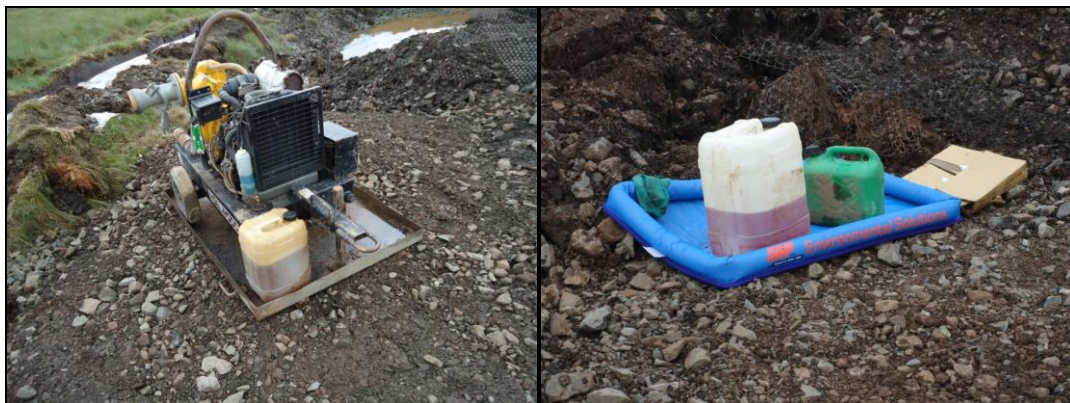
Plate 12: examples of drip trays and bunds
