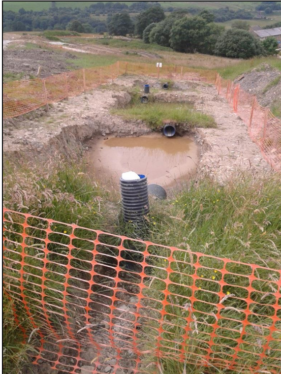
Plate 5: Typical lagoon and flocculent station
